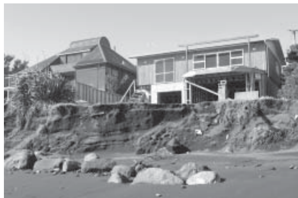
A combination of high tides, large swells and high winds have caused major erosion in front of some properties at Oakura Beach.
