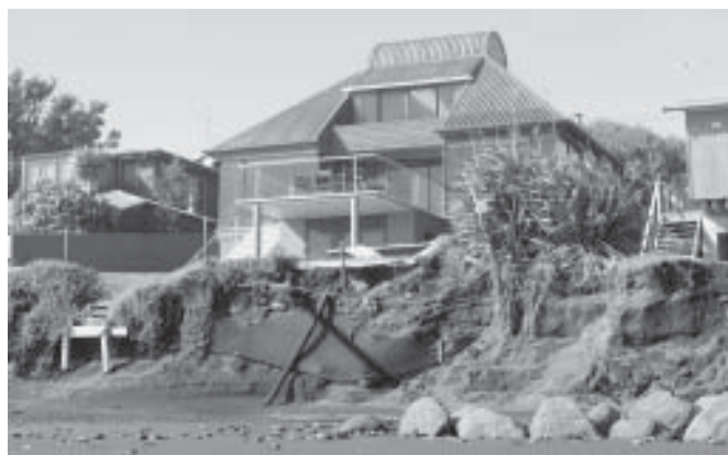
A resource consent has been granted for property owners to build a boulder riprap to help prevent further erosion such as this, in front of 21 sections on the Oakura Beach front.
