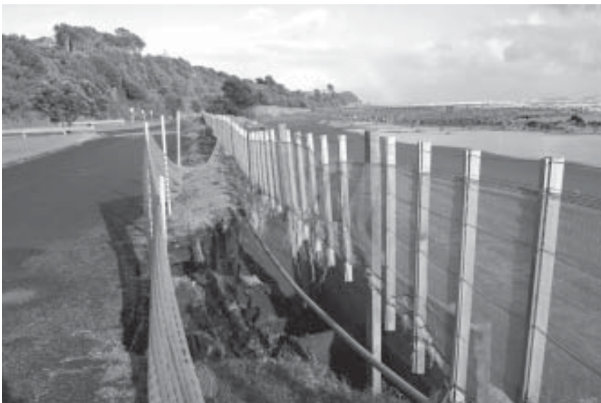
A section of road in the Oakura Beach Camp has subsided and needs attention.
